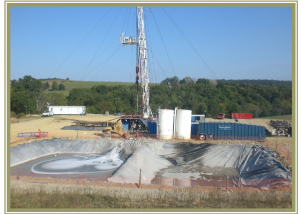
Gas well drilling, 2010
