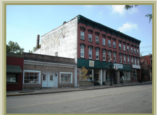
Deteriorated buildings (Steering Committee Photo, 2011)
