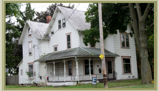
Older homes with maintenance issues (Steering Committee Photo, 2011)
