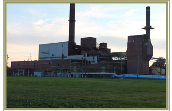
City of Orrville Power Plant (Steering Committee Photo, 2011)
